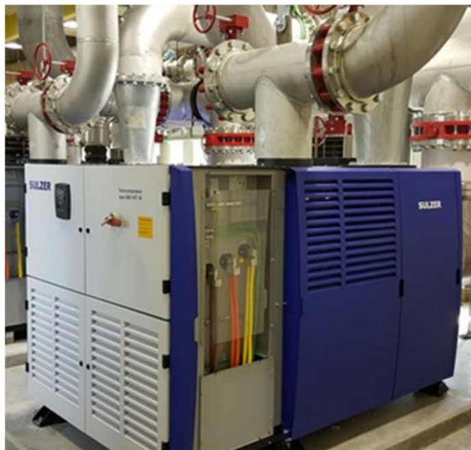
New turbo blowers (manufactured by Sulzer-ABS).
